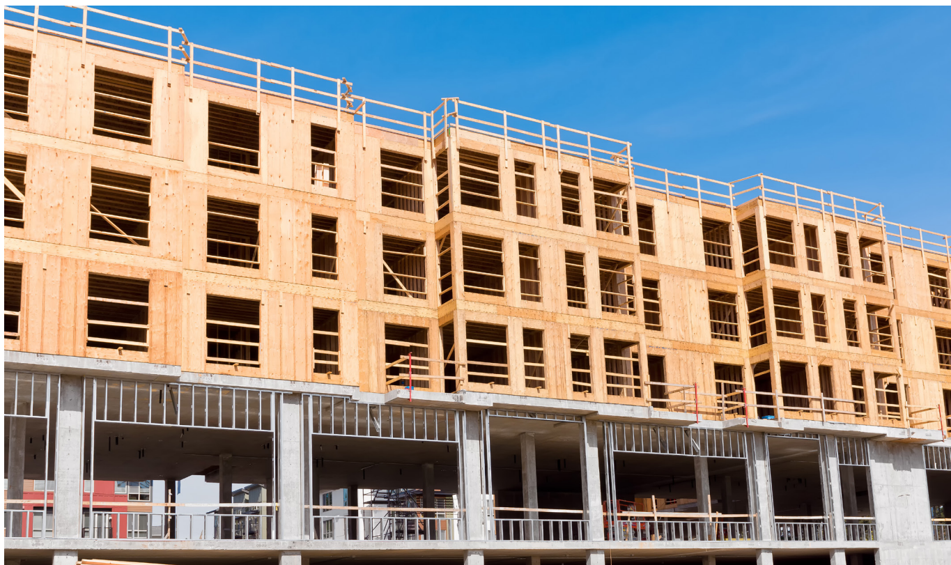
Low-cost housing units using timber under construction | Credit: JohnnyH5
