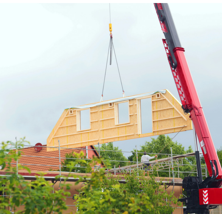
Assembly of a prefabricated timber house | Credit: Gabriele Grassi
